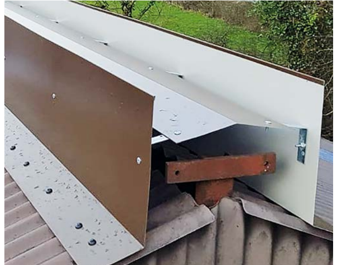
A covered open ridge is an optimum outlet
