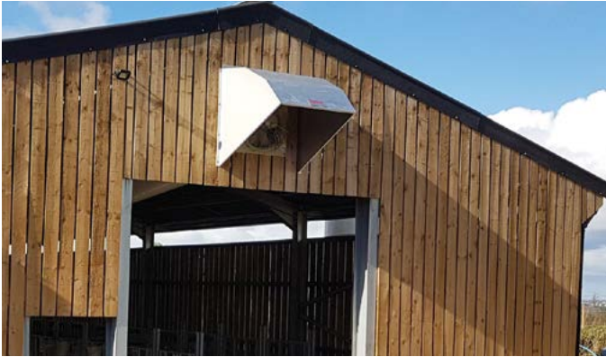
Fans in most sidewall locations benefit from an external cowl to protect the fan and provide more consistent operation
